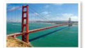
Golden Gate Bridge
